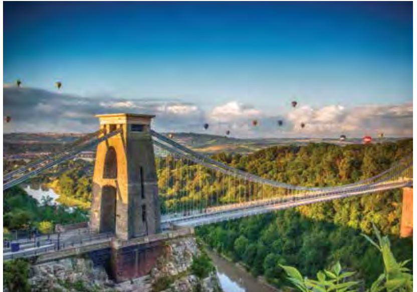
Clifton Suspension Bridge, Bristol
