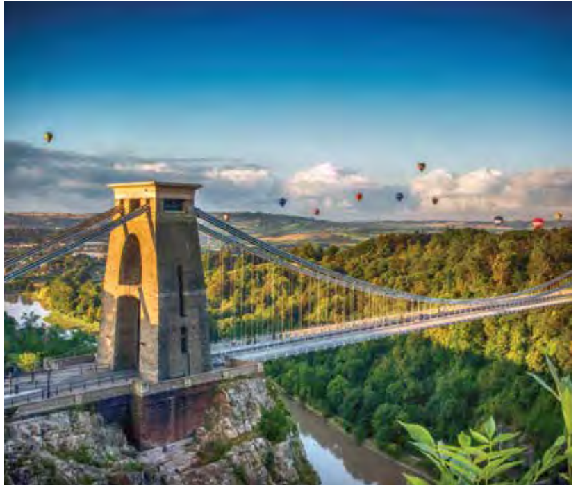
Clifton Suspension Bridge, Bristol
